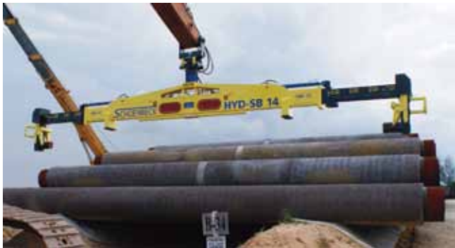
Figure 6. Lift signal inactive.
