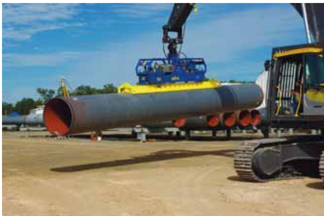
Figure 3. ELiTE 16TD – pipeline construction.
