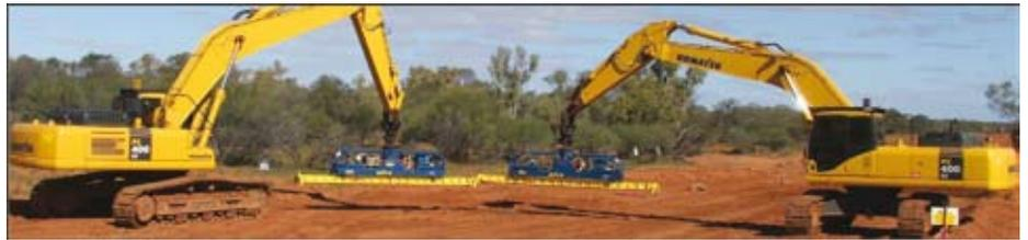
The ELiTE vacuum pipe lifter is a new vacuum pipe lifting concept, capable of operating in some of the world's most inhospitable environments. The simple design and engineering of these lifters enables staff to quickly and easily obtain a sound understanding of the equipment, reducing equipment downtime, which is often caused by operator error.
